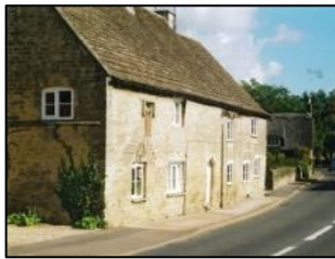
No. 7 Station Road
